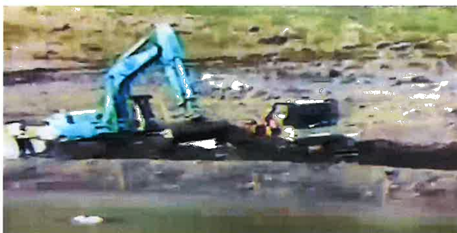
Fig. 23: Previous WCC works underway on client farmland
